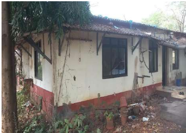
Office Block (Admin Building)
